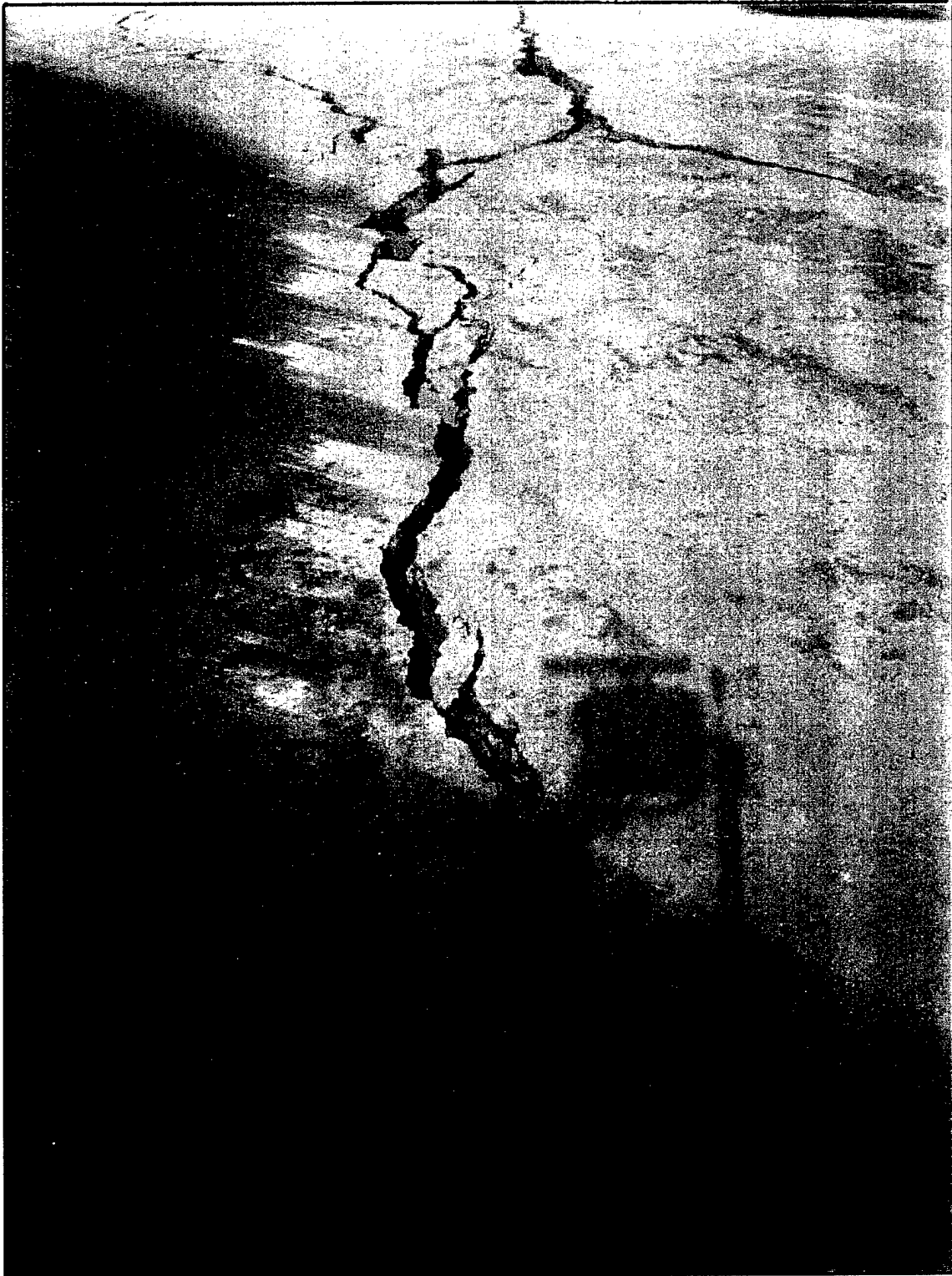
Figure 3-9. Cracks in prepared surface (trailer park) on Rainier Mesa. These cracks formed prior to collapse sink formation.
